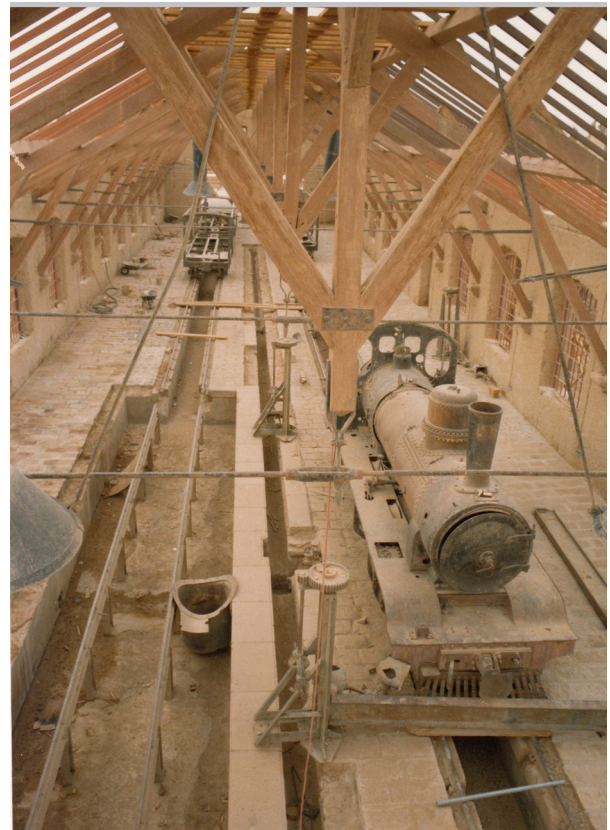
Figure 9: Mada'in Saleh 1985, Hejaz Railway sheds under renovation. Photo: Wright Archive
