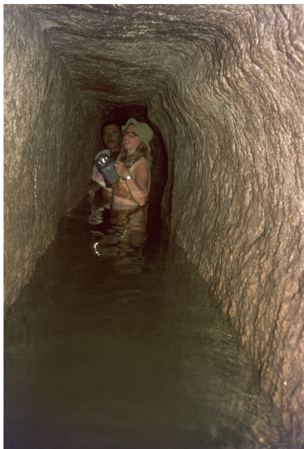
Figure 6: A view inside the tunnel. The regular shape of the tunnel and the smoothness of the walls displays careful workmanship. Photo: the editor 1974.
