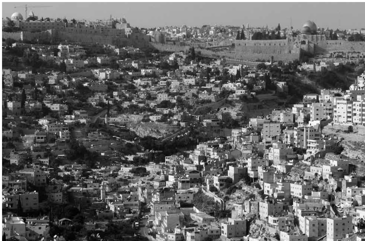
Figure 9: Silwan, the village in which the City of David is located (on the spur in the center of the photo). Photo by Bert de Vries
