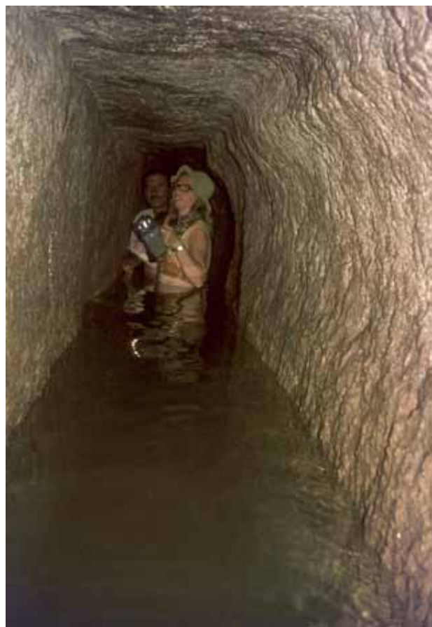
Figure 6: A view inside the tunnel. The regular shape of the tunnel and the smoothness of the walls displays careful workmanship. Photo: the editor 1974.
