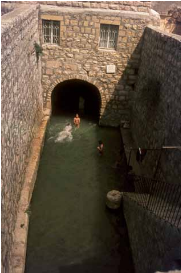
Figure 5: The Pool of Siloam. The tunnel exit is under the right side of the arch behind the standing figure. Photo: the editor 1974.
