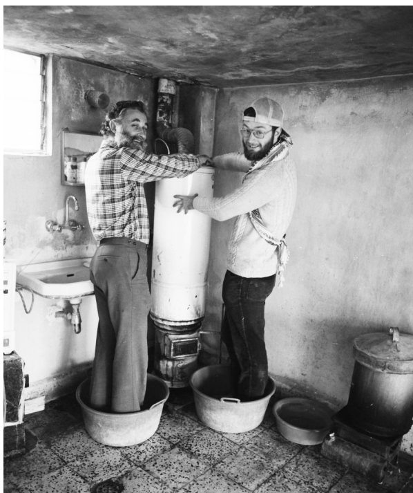
Figure: 9 Ian Edwards and Stephen Bourke at Pella 1985 repairing a hot water service. Image: courtesy Stephen Bourke.
