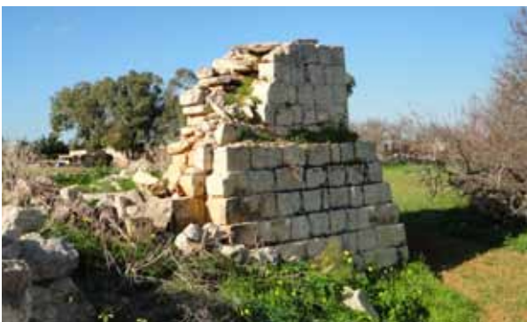
Figure 27: Stepped foundation of a possible Punic monument east of Safi (35° 50.019'N, 14° 29.905'E. Photo: C. Sagona.
